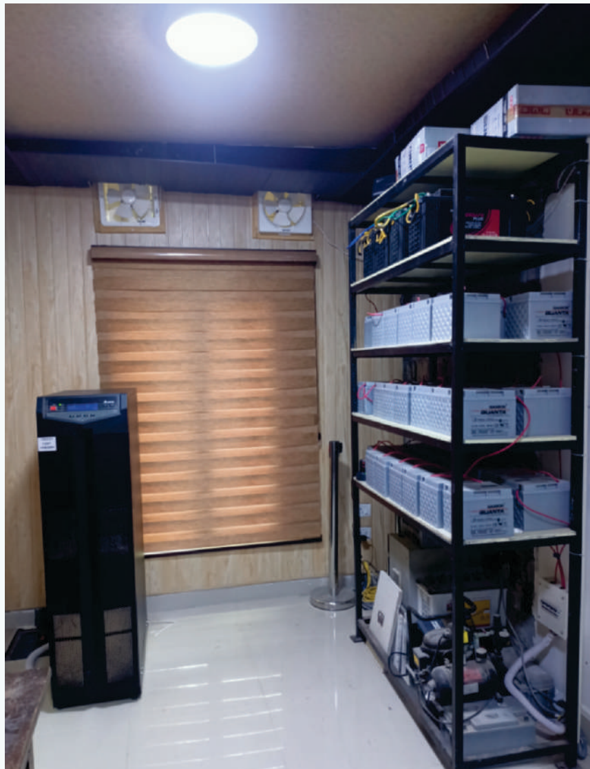
Figure 49. The 20kVA UPS system installed in the electronics lab.
