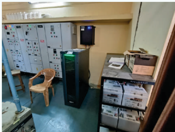
Figure 46. 30KVA UPS and control panel installed at 40-inch coating plant.
