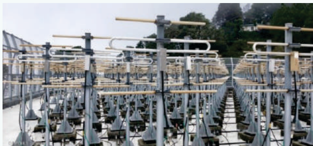
Figure 62. (Top) In-house production of spare TRMS; (Bottom) Integration of in-house design, fabricated folded-dipole in one sub array of ASTRAD active aperture.
