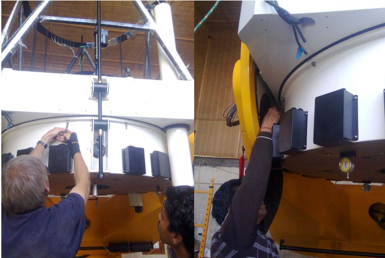
Figure 25: tightening the bolts joining the mirror cell and the centre piece
