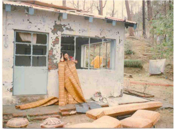
A scientist's house on-campus with broken windows, door, roof, and plaster from the hail storm (May 7th, 1998).
